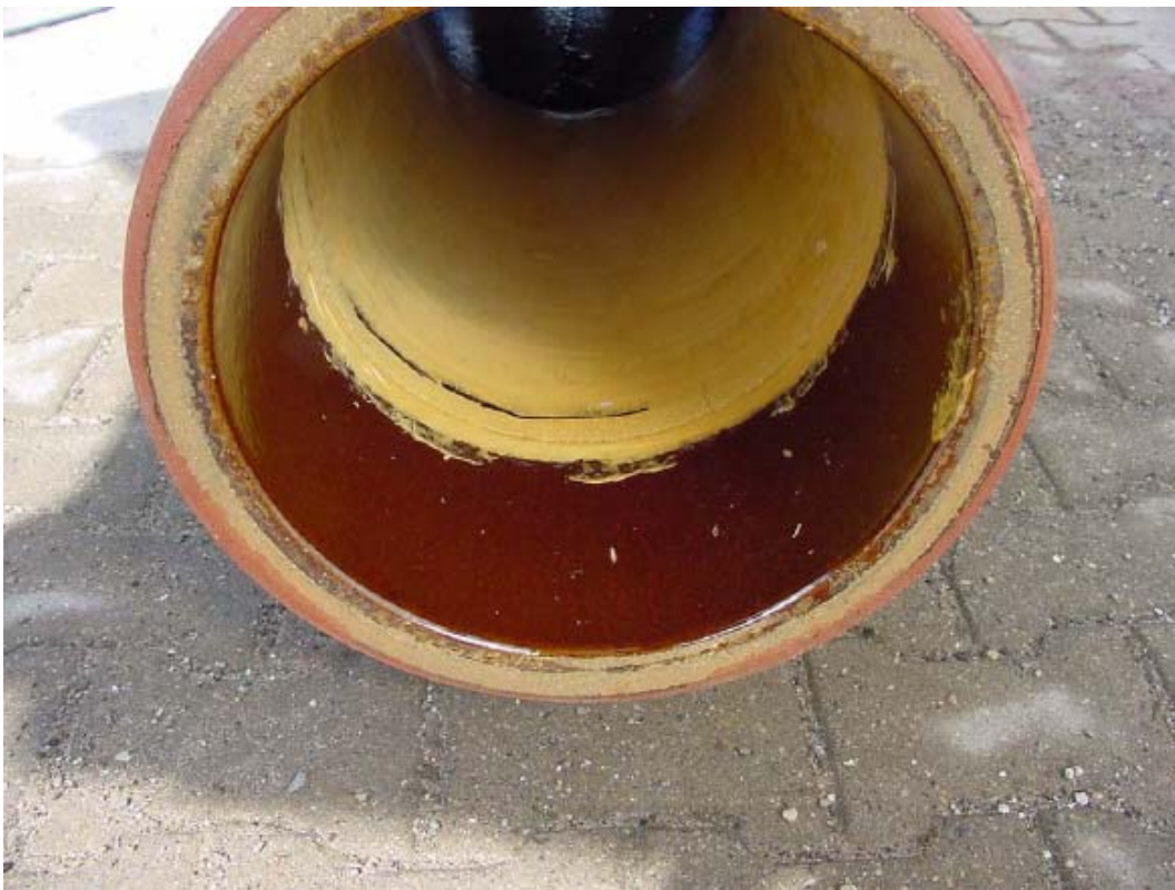
Picture 6: epros patch liner H1263-1.1 prior to jetter test
